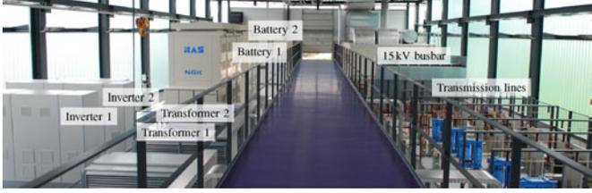
Fig. 2. Technology centre of Younicos AG in Berlin with NaS Batteries, 500-kW inverters, transformers, transmission lines, and 15-kV busbar.
